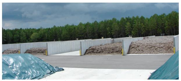
Vista Organics Recycling Facility's aerated static pile system
